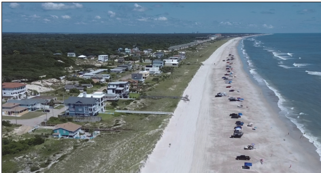
Photograph 2.1: Northward looking view at R-59 (Burney Park) on 27-August-2023.
