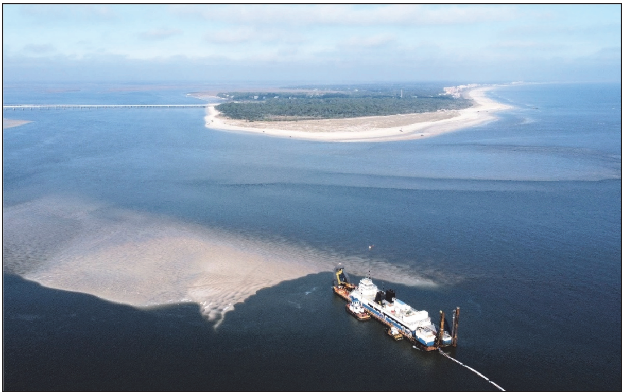
Photograph 1.2: View northward toward South Amelia Island of the Dredge Savannah excavating the shoal borrow area in Nassau Sound. (30 Dec. 2021)
